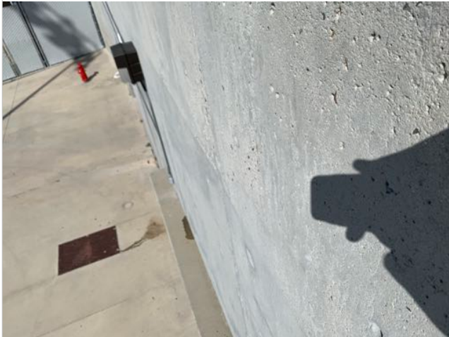
WATER DRAINING THROUGH WALL AFTER MEMBRANE CUT
