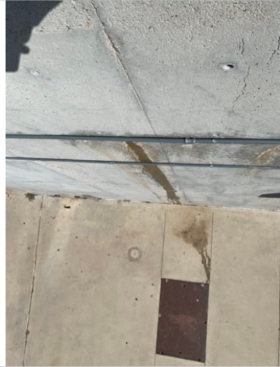
7 WATER DRAINING THROUGH WALL AFTER MEMBRANE CUT
